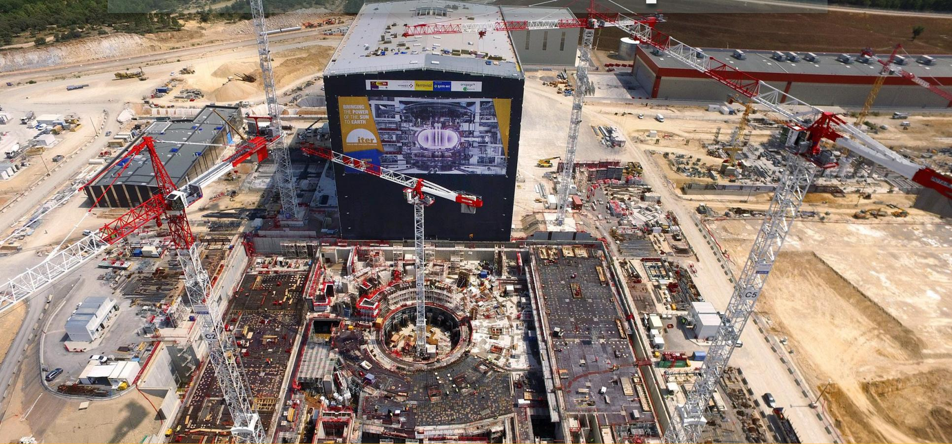
Resting on 493 seismic pads, the reinforced concrete “B2” slab bears the 400 000-ton Tokamak Complex. Concrete casting of the B2 slab was finalized on August 27, 2014. Diagnostic Building (right): B1 level slab and walls/columns now complete; Tokamak Building (centre): completion of the BioShield wall B2 level. Start of the B1 slab on 26 April 2016, and construction of interior walls/columns is on-going. Tritium Building (left): steel reinforcement on B1 level.
