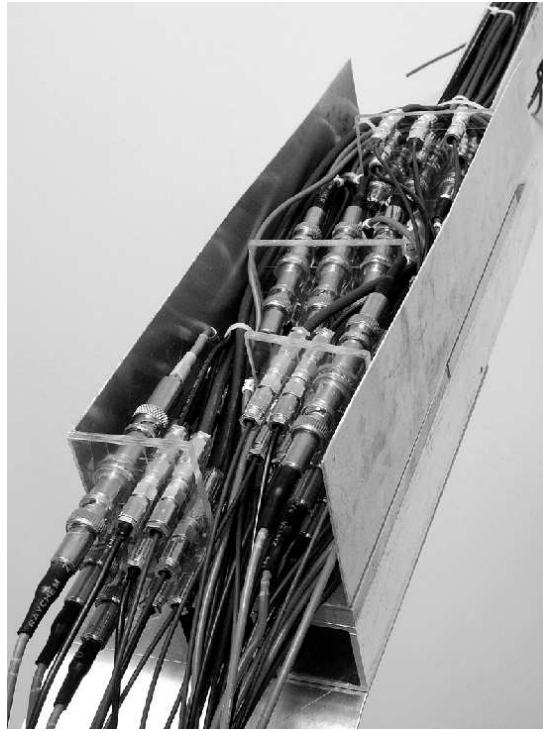
Figure 1.14: T0 patch panels inside the duct on the top of the muon absorber.
