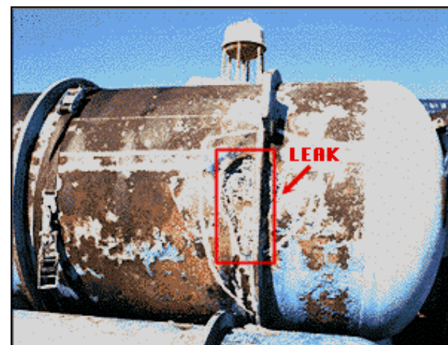
Cylinder Leak
